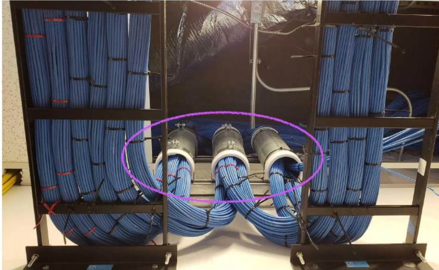
Chase pipe/conduit sleeve example
